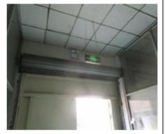
OB1: The factory's 80% emergency exits were installed with rolling doors
